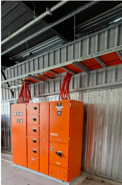
Evaporative plant works – Existing Market carpark level 2
